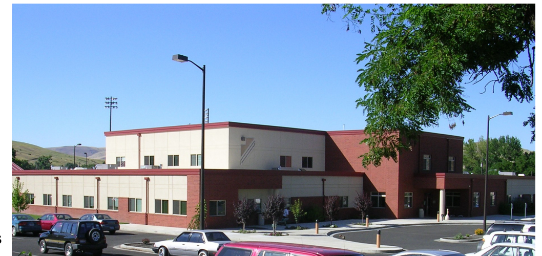
The Nimiipuu Health Clinic in Lapwai, ID, houses the Health and Wellness Center
